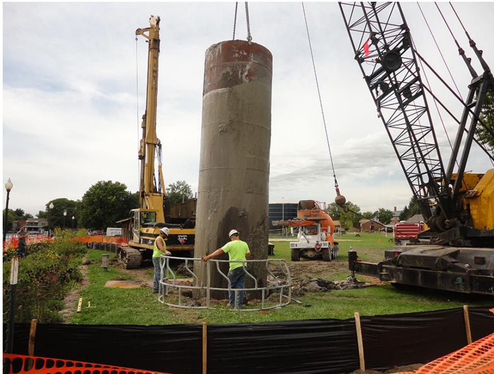
Nearly 80 tons of concrete were used to construct a base that is nearly 7 feet in diameter and 30 feet deep! Such a monumental base is required because, at 160 feet, this flag pole is the tallest in the State of Michigan!
